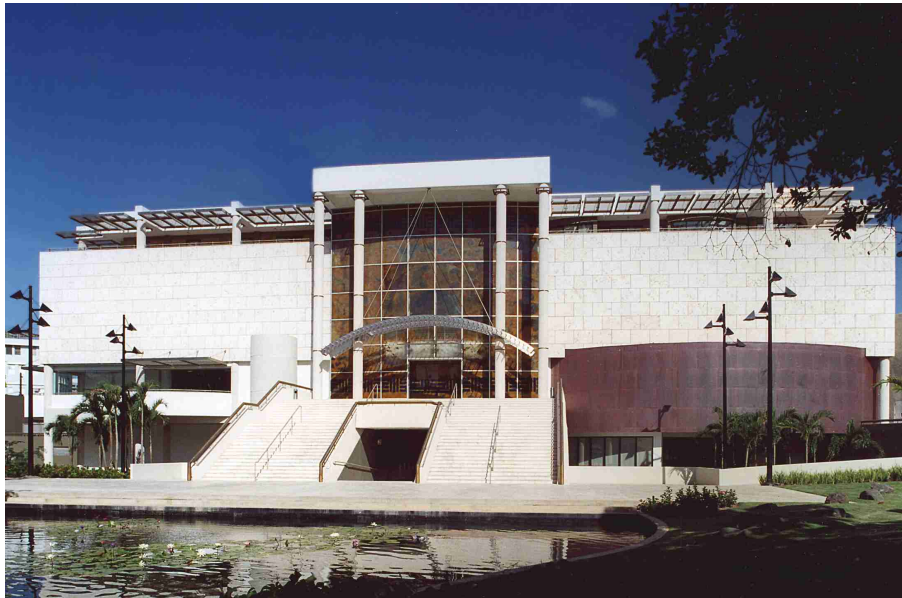
Exterior - Rear Facade
